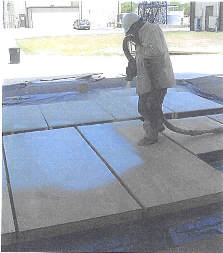
Figure B-1. Application of SPF.
