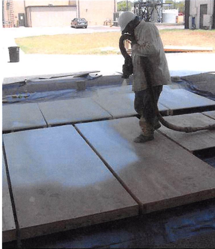
Figure B-1. Application of SPF.
