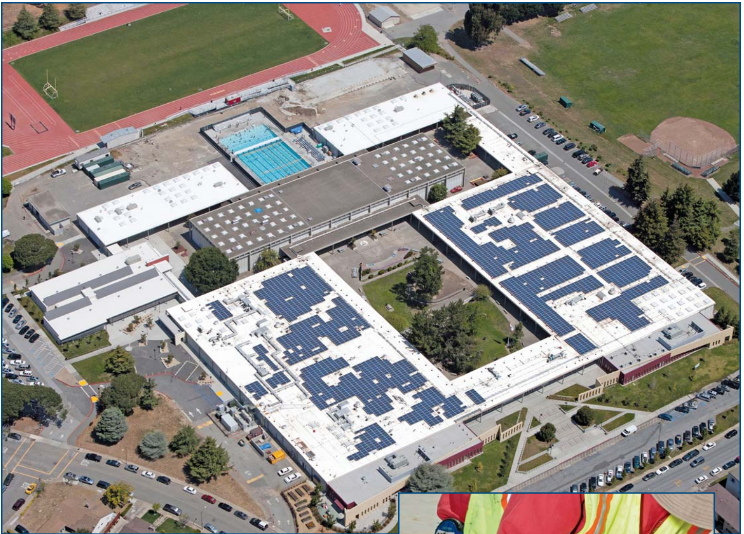
Photo 1 – White EPDM roofing membrane serves as a high-performance foundation on a multifacility reroof project for the San Mateo Union High School District that featured more than 2,500 photovoltaic panels installed atop three California high schools.
