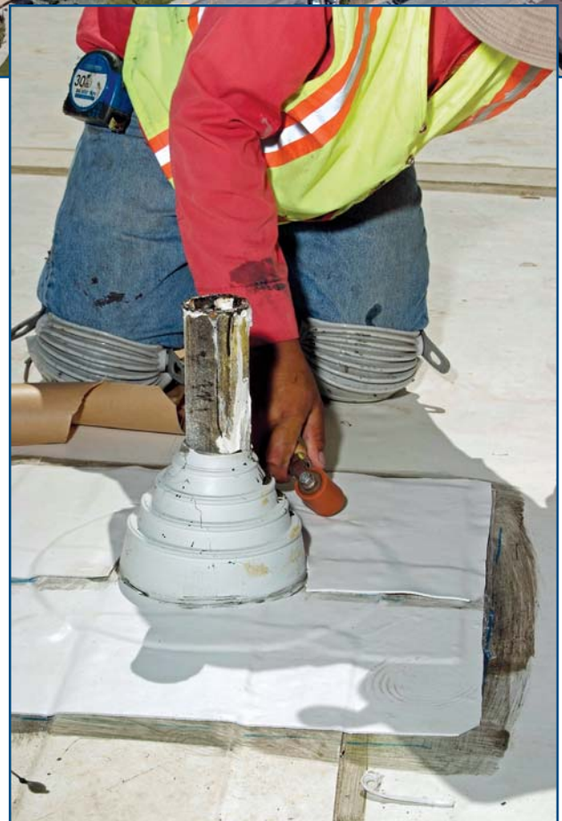
Photo 2 – Customized white EPDM target patches and boots used around the stanchions to support the PV panels helped expedite the installation process.
